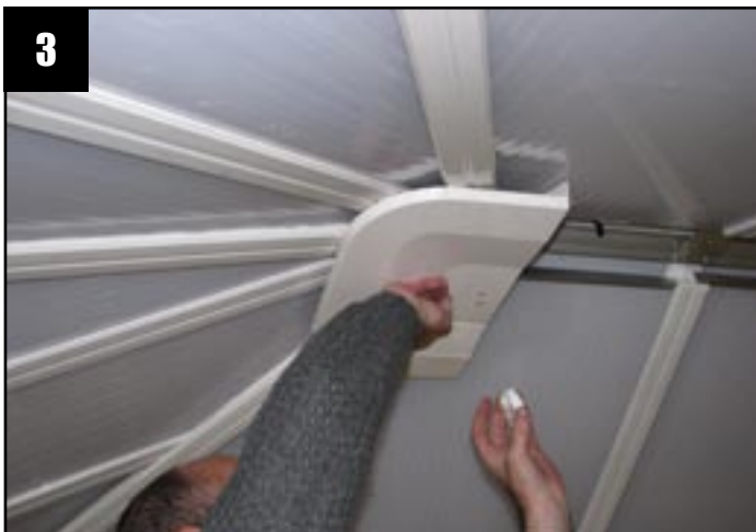
Offer the internal radius end capping over the threaded rod. (The rod may require cutting to length).
