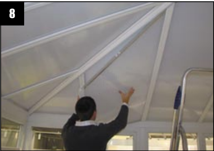
Install panel position 4 with 'T' section.
