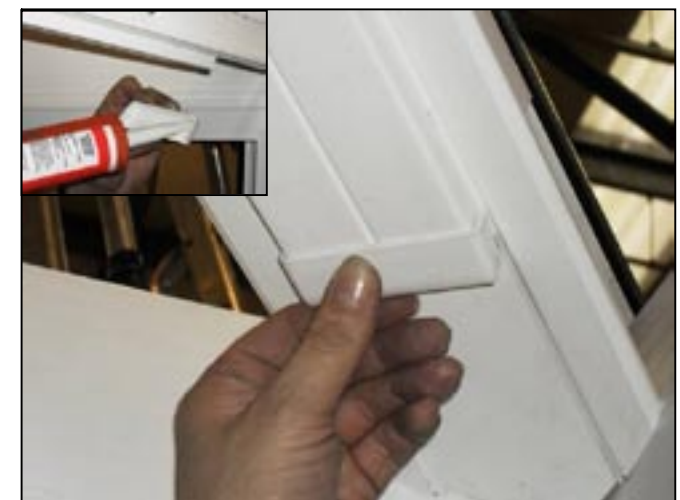
10. Silicone and fit bolter end cap. •BLBC001/1 – Transom •BLBC001/2 – Georgian Hip •BLBC001/3 – Victorian Hip
