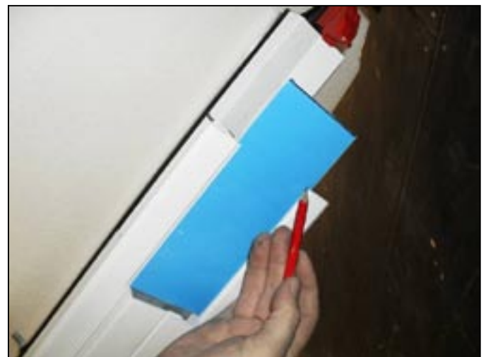
20. Mark the infill plate at the end of the L sections and square cut across. Re fit and attach bolster end cap (BLBC001/1,2 or 3) as per the bottom of the bolster hip bar. (See step 10).
