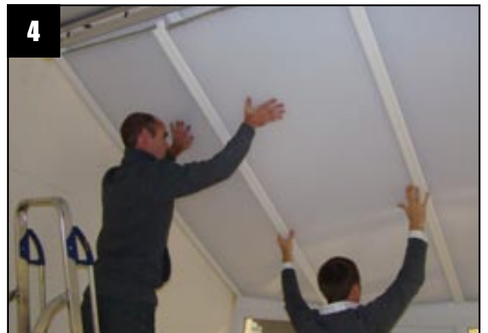
Whilst holding the first panel in position, locate the second panel and 'T' section into position as shown. (Fig 1)
