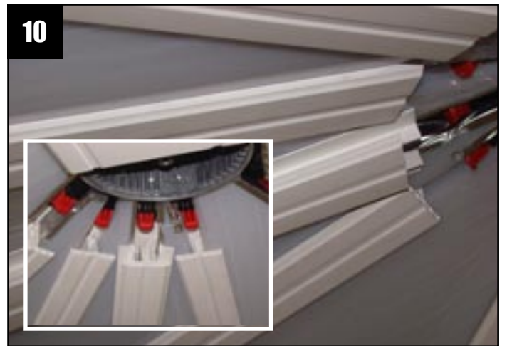
Image shows the angle trim in position at the radius end.
