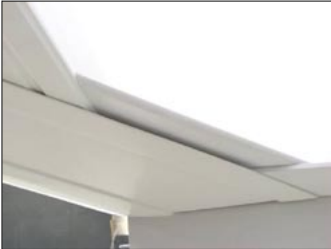
•Finished trim shown in position.
