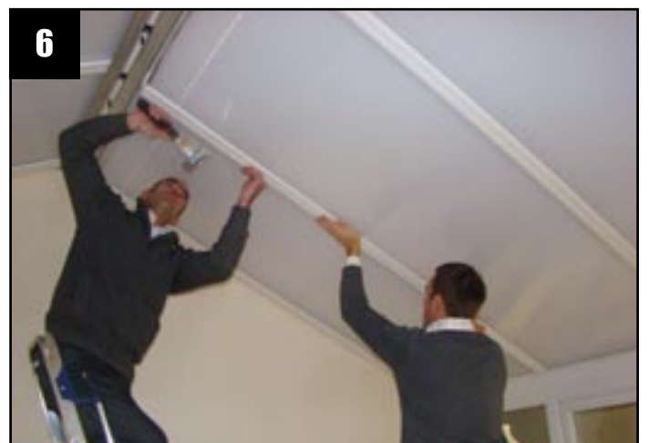
Fix central 'T' section into the glazing bar undercladding. (Fig 4)
