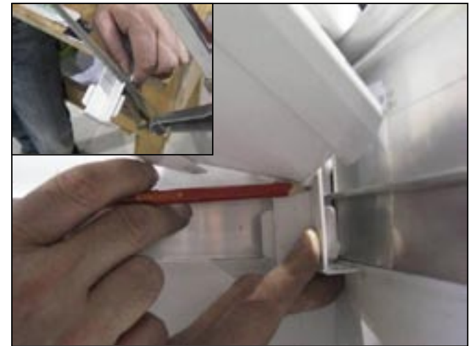
8. Slide Fascia corner behind bolster and mark using lower edge of bolster infill plate. Cut corner to this line.
