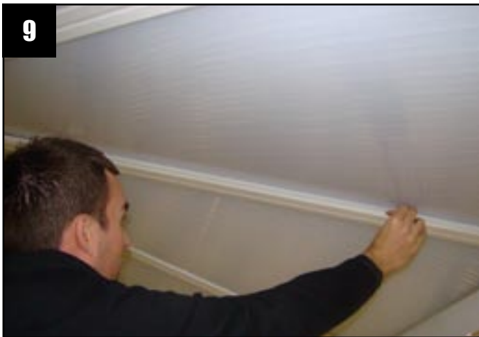
Roll in the angle trim and press firmly into position (the tape sticks against the polycarbonate).
