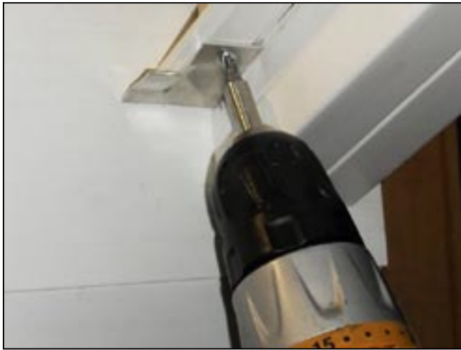
15. Using the self drilling screw provided, fix bracket into L sections hard up against the bolster as shown.
