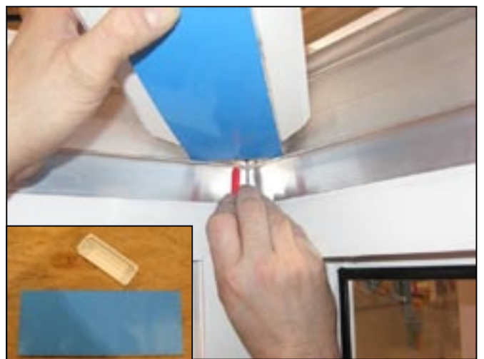
4. Using infill kit (BLBC001) hold plate (BLBC001/2) in centre of hip bar and mark position where eaves beams meet.
