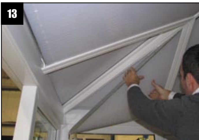
Slide fit panel position 12 into 'T' section as shown and hold
