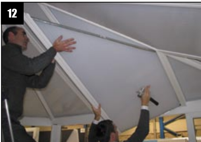
Offer up panel position 9 and 'T' section and slide fit into the jack rafter 'T' section as shown above. Continue with panel position 10 and position 11.
