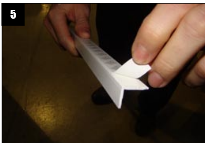
Trial fit the angle trim into position, remove the adhesive backing.
