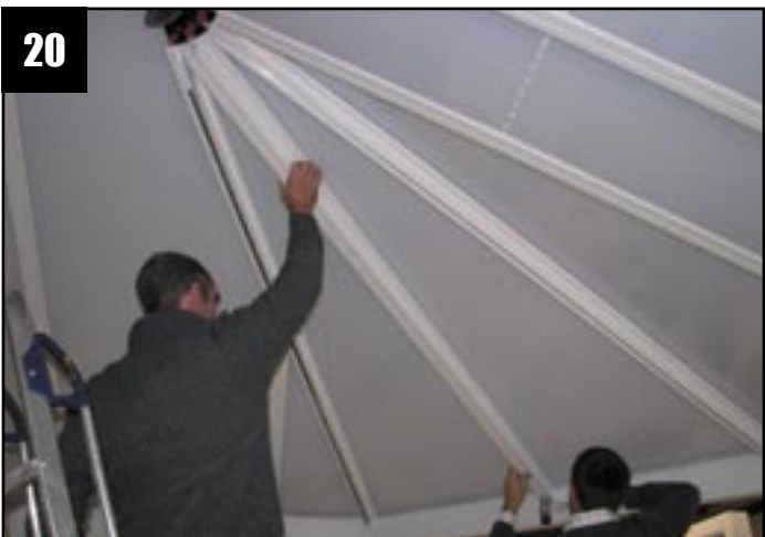
Fit the centre 'T' sections
