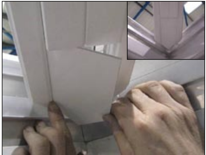
6. Fit cut down plate between L sections. The plate should sit in the channels running down the section.
