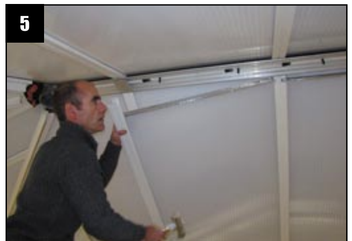
5 Offer panel position 2 with the 'T' section attached and fit as per panel position 1.
