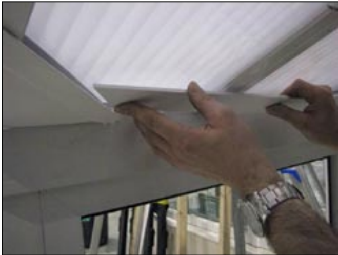
6. Tuck BLDC into valley cladding.
