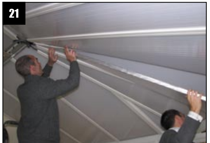
Slide fit the panels into the 'T' section, hold in position and fit the hip 'T' section.
