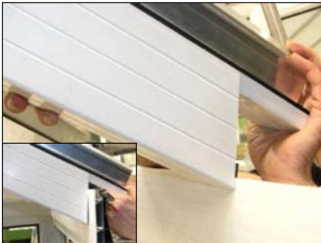
11. Fit transom bars (bolstered bar shown).
