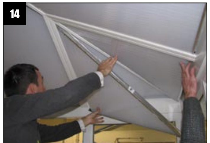
Slide fit panel position 13 into 'T' section and hold.
