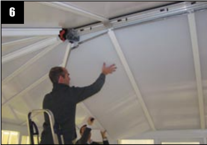
Install panel position 3 with the 'T' section.
