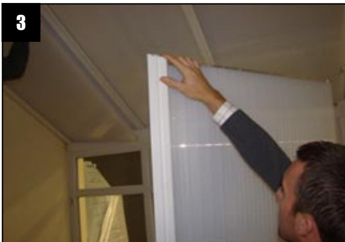
Locate 'T' section on to the second panel.
