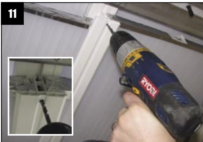
Drill the hole approx 15mm from the end of the 'T' section.
