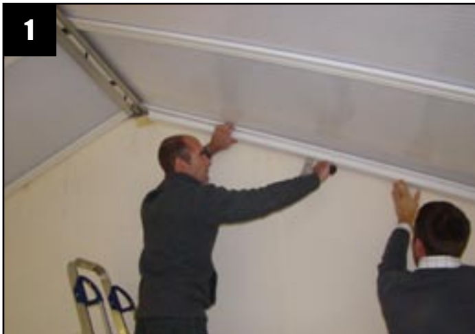
Fit the starter bar 'T' section by clipping up into the glazing bar undercladding. 'T' section should be tight up against the fascia board.
