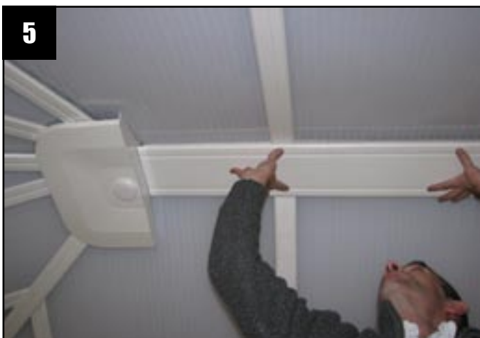
Measure, trim and push fit the ridge undercladding into place.
