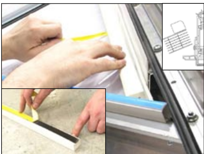
13. Mark and cut to length 08586W1 (20mm x 25mm). Peel back protective film off tape and secure down the lengths of the lower layer of polycarbonate.
