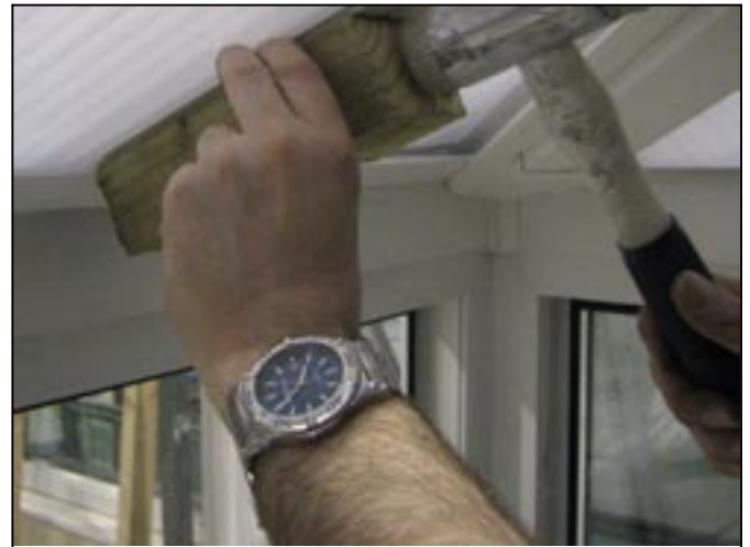
7. Using drift, knock BLDC into position to secure.
