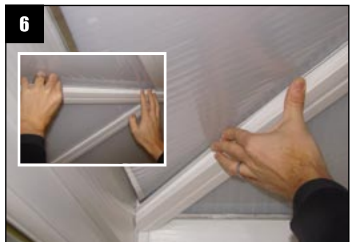
Roll in the angle trim and press firmly into position (the tape sticks against the polycarbonate).
