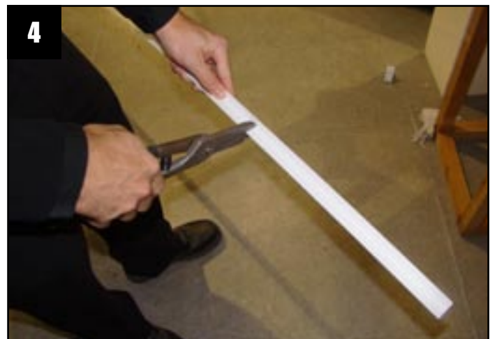
Cut the angle off with snips (shown) or hacksaw.
