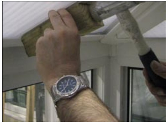
18. Using drift, knock BLDC into position to secure.
