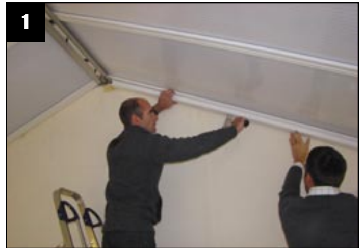
1 Fit the starter bar 'T' shaped cladding section by clipping up into the glazing bar undercladding. 'T' section should be tight up to the fascia board.
