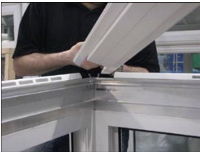
1. Fit bolster bar into the socket at the radius end. Then at the eaves, fit by rocking over to the side and feeding over the eaves then rock over the opposite way.
