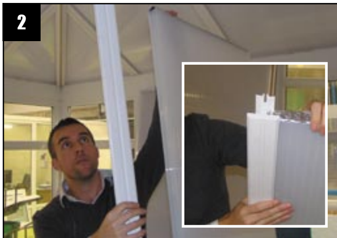
2 Locate 'T' section on to the internal panel as shown.
