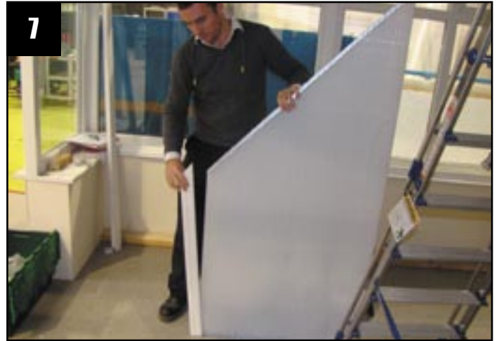
Locate 'T' section onto the internal panel
