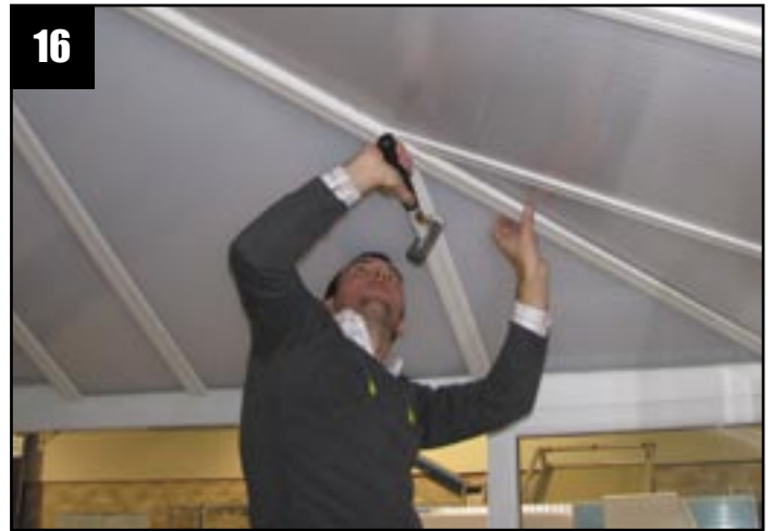
Fit the hip 'T' section.
