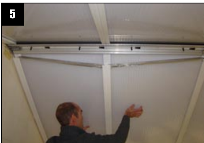
Lower the first and second panel as shown hinging around the fitted 'T' sections. Rotate central 'T' section to 'receive' both panels, locate and push up. (Fig 2 & Fig 3)
