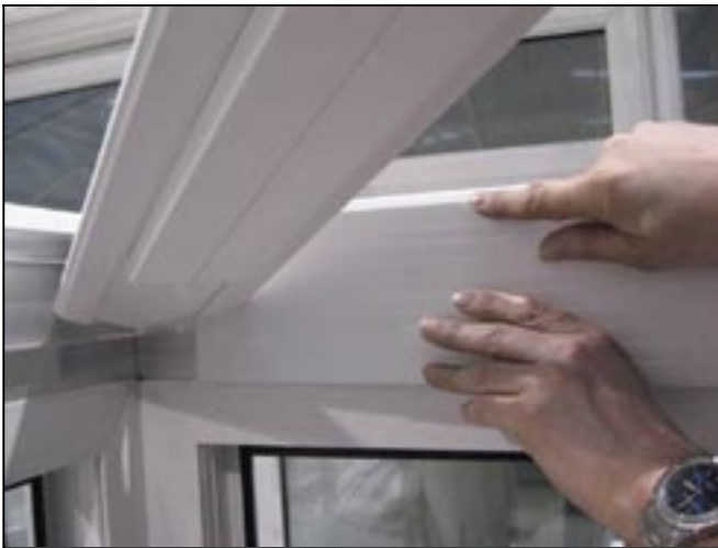
7. Fit eaves fascia at this point. Slide eaves fascia in behind hip bolster bar. Leave a slight gap between adjacent eaves beam for fitting corner.
