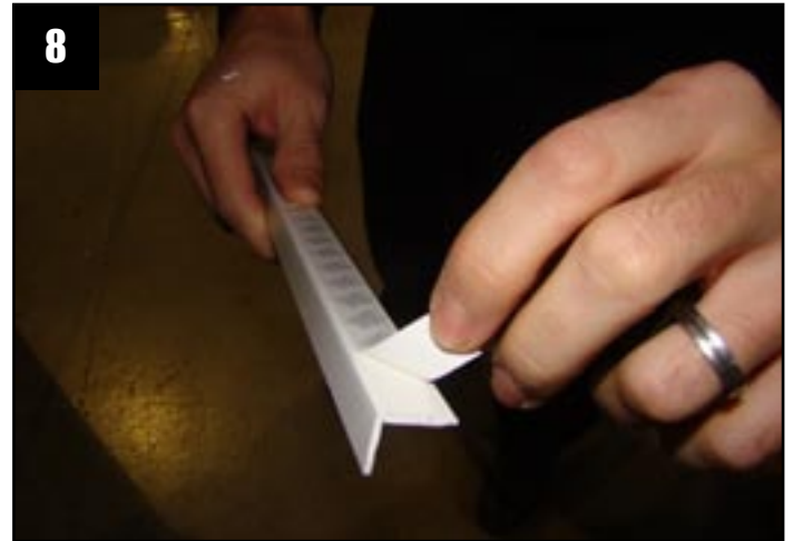
Trial fit the angle trim into position, remove the adhesive backing.
