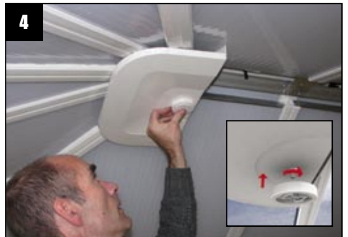
Fix the threaded disk and clip fit the disk cover plate.
