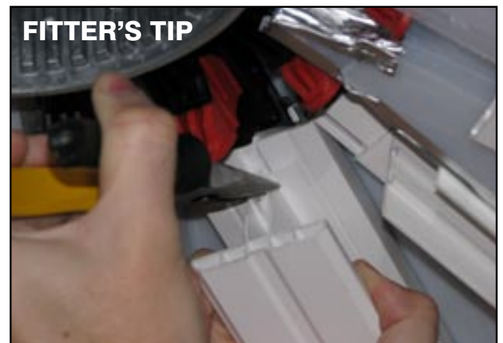
To remove the 'T' section - Squeeze the 'T' section legs together as shown and pull down.
