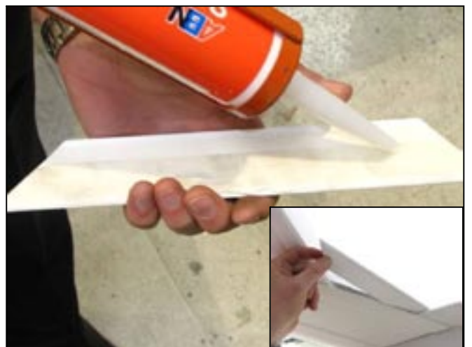
4. Apply small bead of silicone to underside of architrave and carefully fit along valley undercladding.
