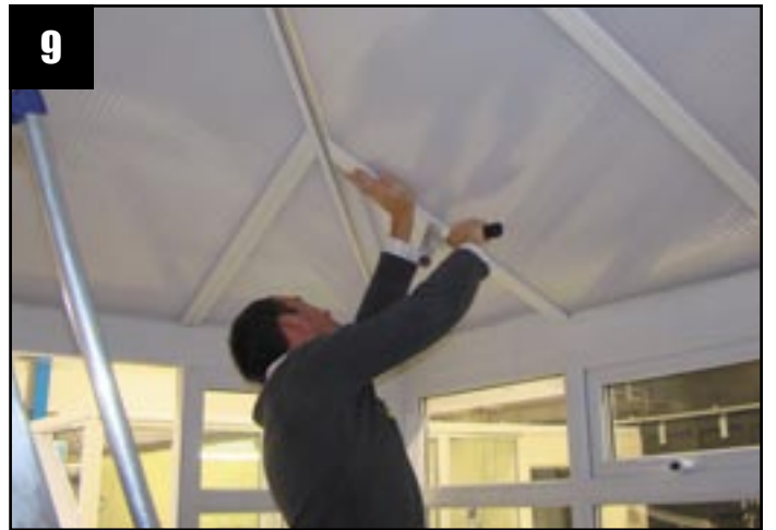
Clip fit the 'T' section onto the glazing bar undercladding as shown
